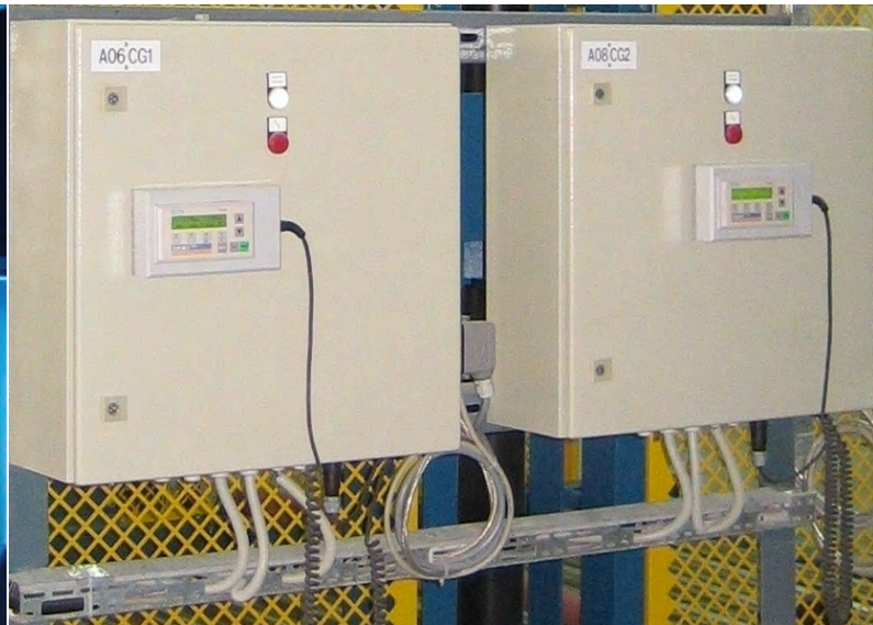
Control cabinets for guiding devices with movable operator panel
