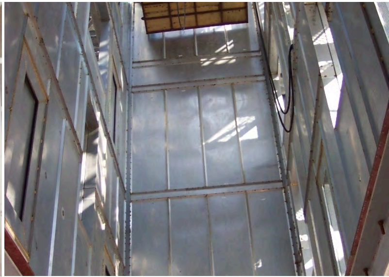
Insulation plates arrangement
